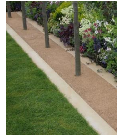
Self binding gravel in warm, pale tone edged with poured concrete strips – 120mm wide and polished
