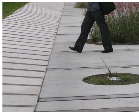
Brushed concrete footpath
